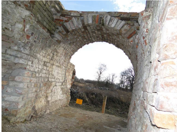
Photo 10 View of the repaired vault at the front wall of the barge from the outside
