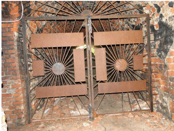
Photo 28 View of corroded steel elements
