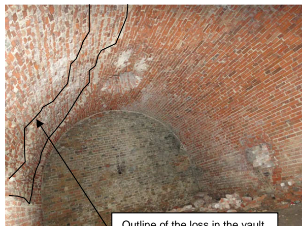
Outline of the loss in the vault at the depth of the whole brick
